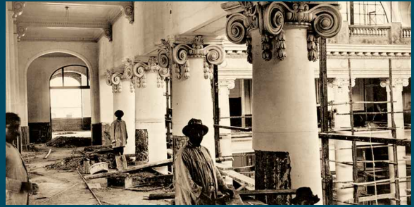
Construction of Head Office.
